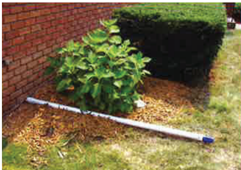
BEFORE Discharge Pipe extending Across Landscaping.
