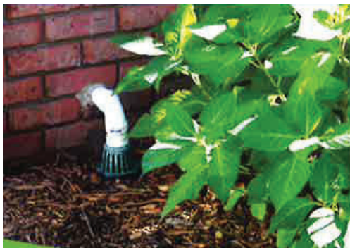
AFTER Discharge Pipe buried, extending unseen into yard.
